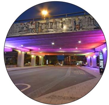
Gosford Street Underpass Coventry, England
