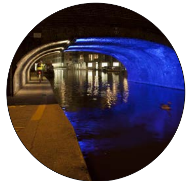
Regent's Canal Tunnel London, England
